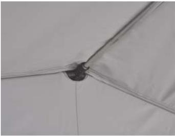
3. Fit apex ridge pole to black 5 way fitting and to top of centre upright pole through eyelet. Peg and tension with guy rope.
